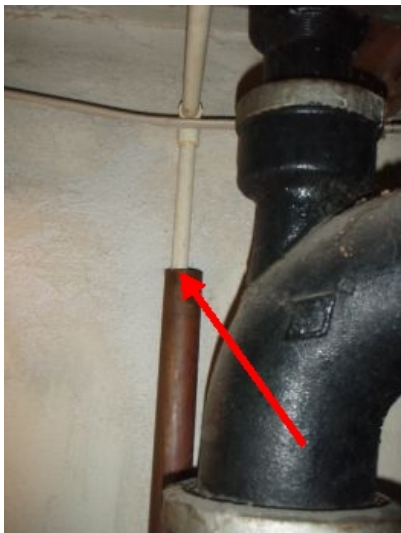
Possible Cross Connection - No Air Gap Between Backwash and Drainpipe
