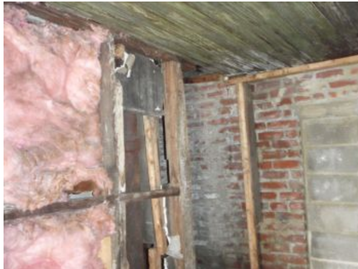
Temporary Supports in Garage
