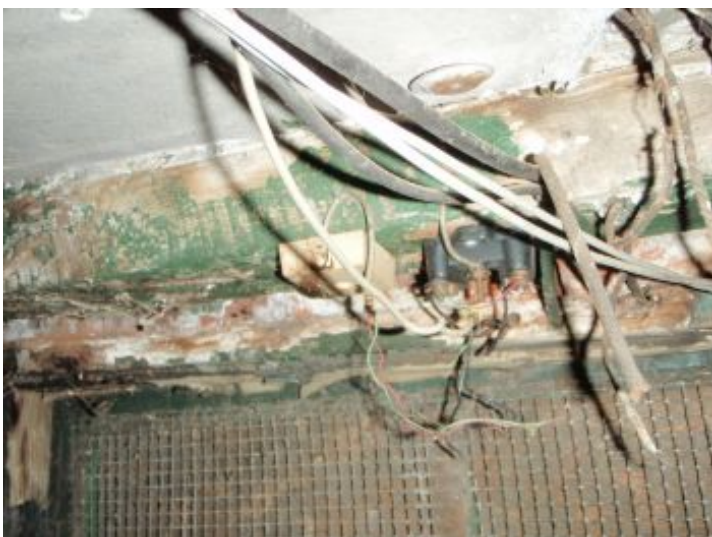
Rotting Window Header
