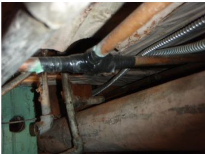
Leak at Supply Line in Basement
