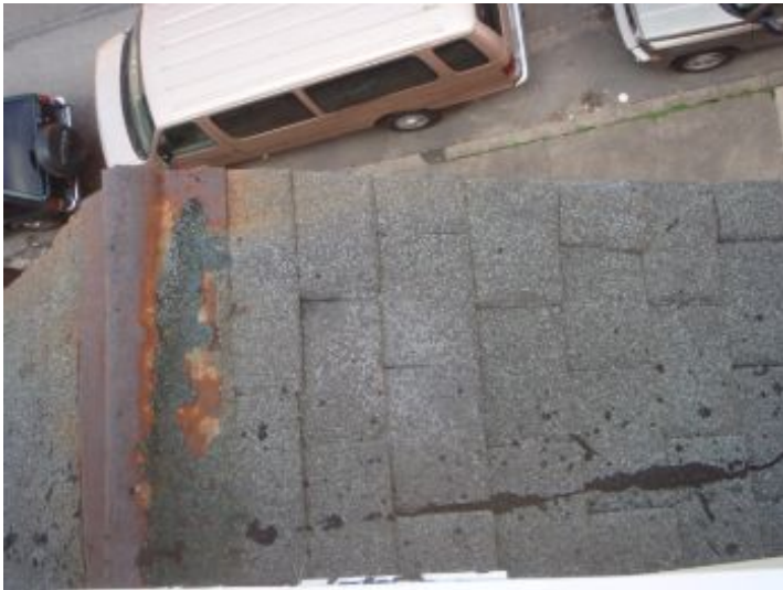
Damaged Dormer Window Roof
